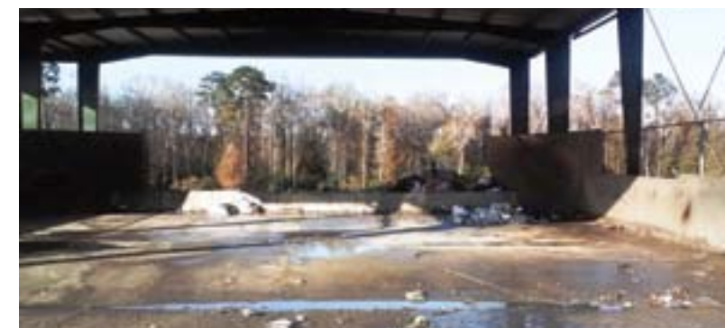
A well-used solid-waste transfer station needing to be upgraded to better manage standing water and garbage leachate.
