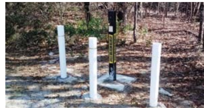
A new groundwater monitoring well placed next to a wetland area in South Carolina to monitor groundwater flow from an adjacent landfill.
