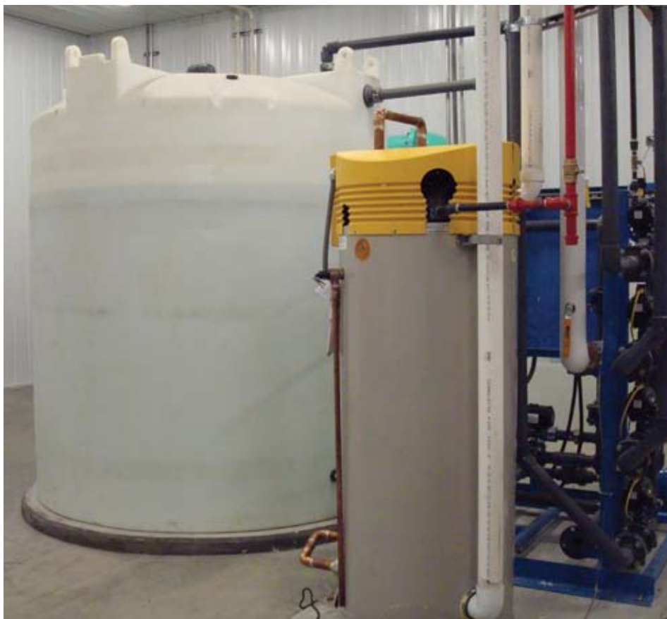
Photos courtesy of Rapid Valley Sanitary District.
