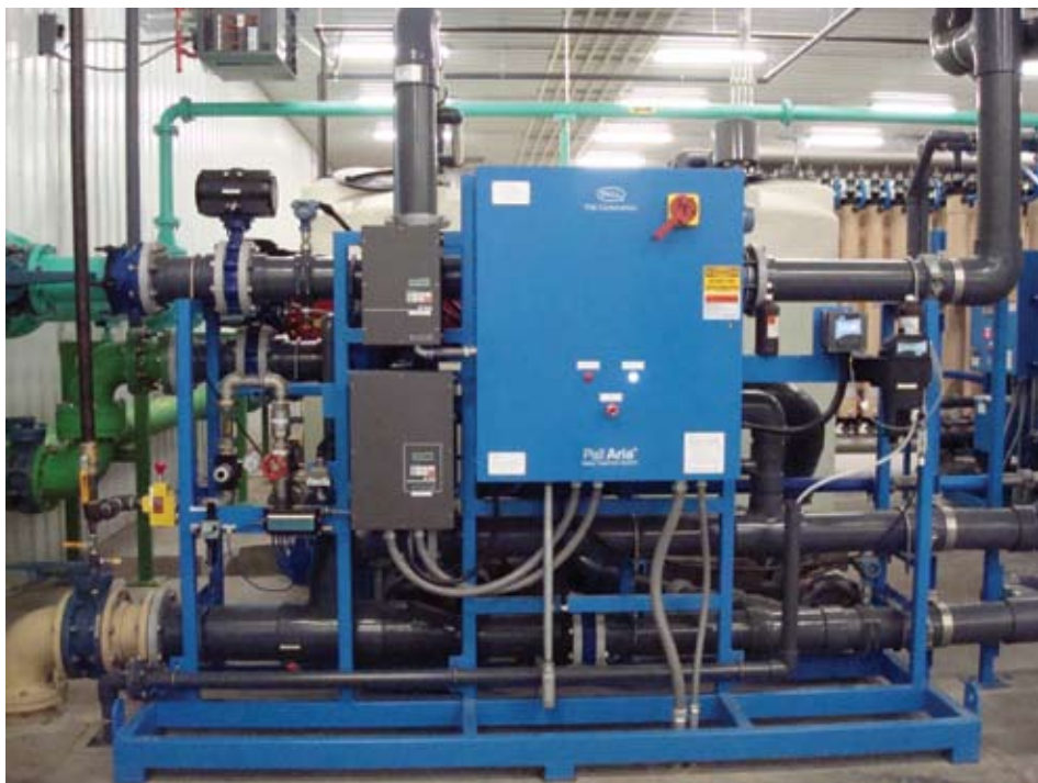
Rapid Valley’s new treatment equipment.
